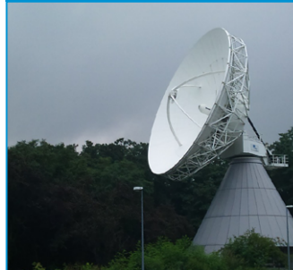
통신기기 Communication Equipment
